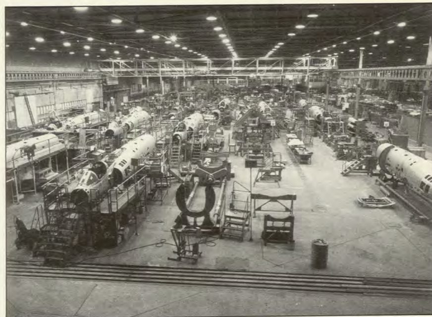
Fuselage production at Government Aircraft Factory at Fishermens Bend, Melbourne (M. Susans).
