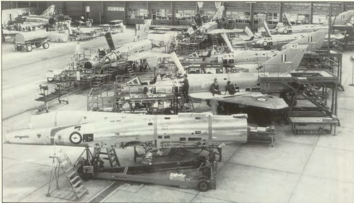
Final assembly line of the Mirage at the Government Aircraft Factory, Avalon. (M. Susans).
