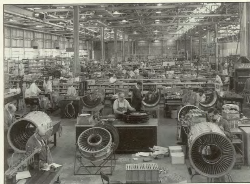
Mirage (Atar) Engine Assembly Line at Commonwealth Aircraft Corporation at Fishermens Bend, Melbourne (M. Susans).
